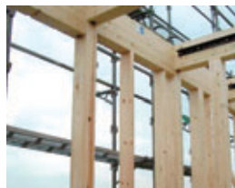
Laminated wood posts made from domestically sourced Akita cedar
